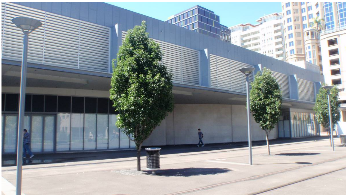
Figure 5: View of the existing substation from the UPN level.
