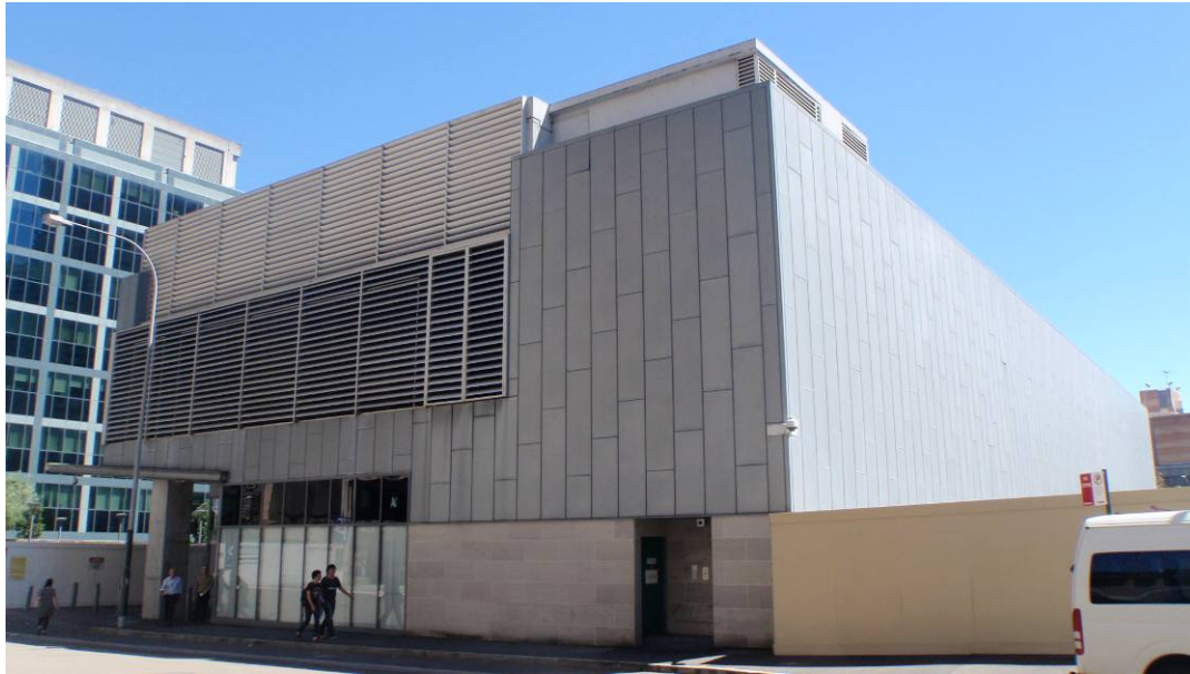
Figure 6: View of the substation from the south on Thomas Street.
