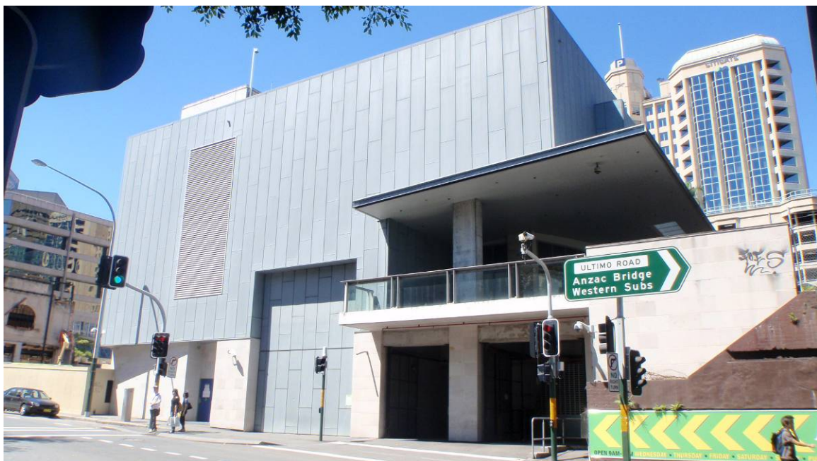
Figure 3: View of the northern elevation of the substation showing existing vehicle access.
