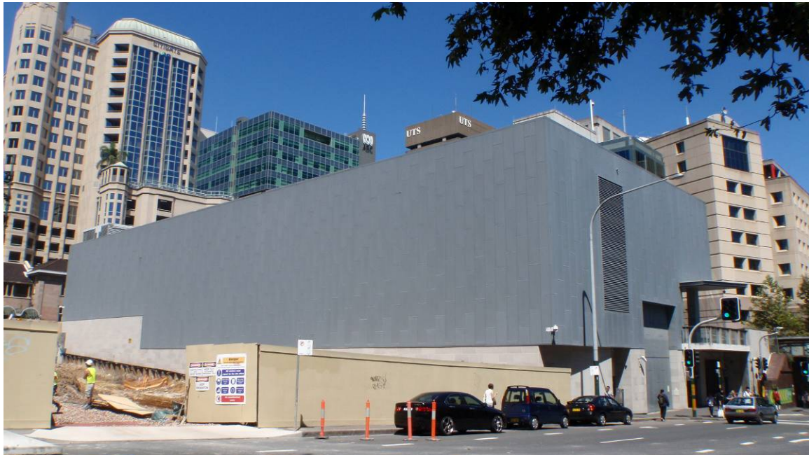
Figure 2: View of the substation from the north east on Ultimo Road.
